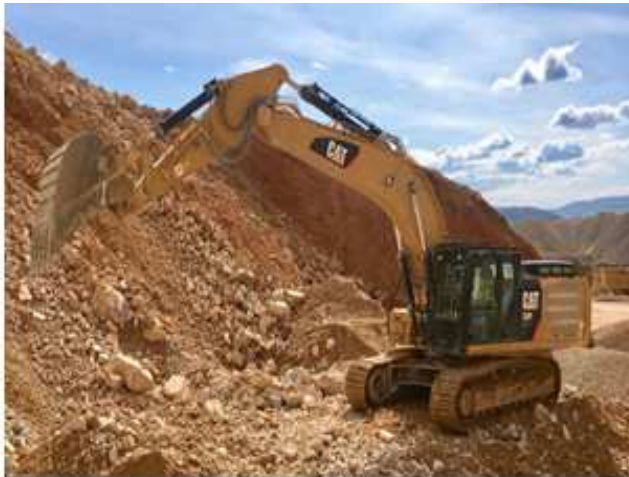
Tracked excavator CAT336F
