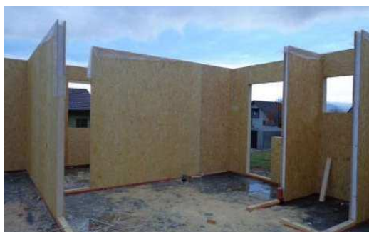
Figure 5 The construction system of Structural Insulated Panels (SIPs)
